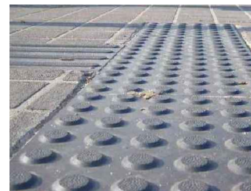
REFERENCE IMAGE TYPICAL BLISTER PAVING
